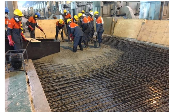
Mozal Reduction Precast Slab Repair
