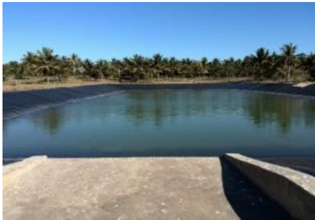
Excavated Water Reservoir in Chicungussa
