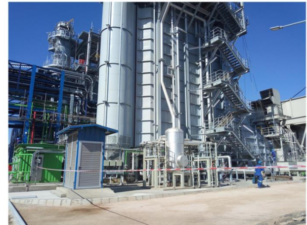
Project of Combined Cycle Gas Thermal Power Plant in Maputo
