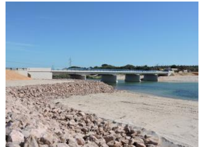
Rehabilitation of the Inharrime Bridge and Slope Stabilization
