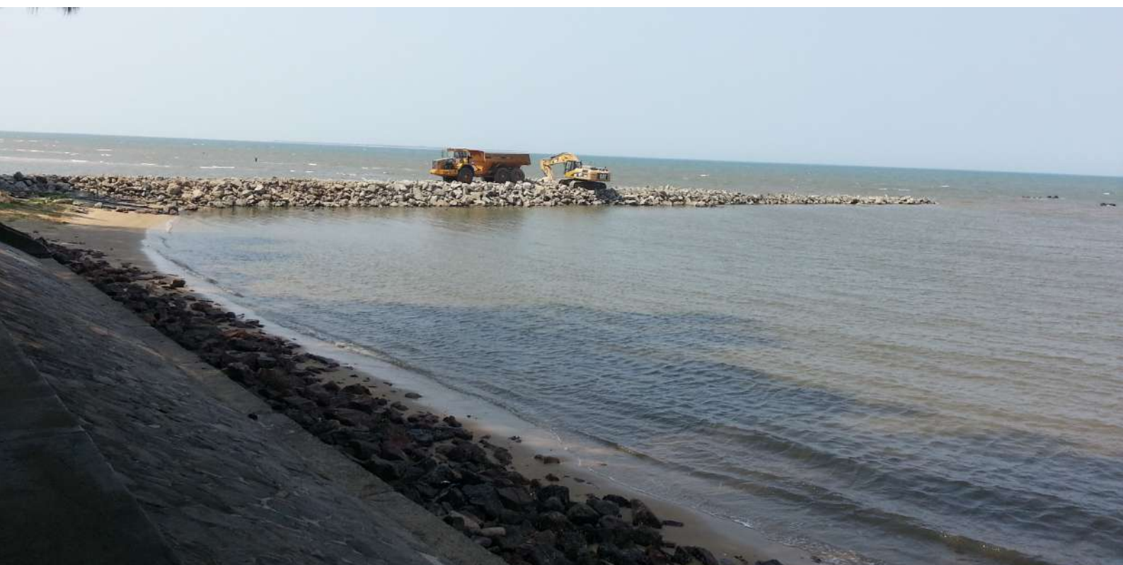
Coastal Protection Infrastructure Improvement Works – Maputo
