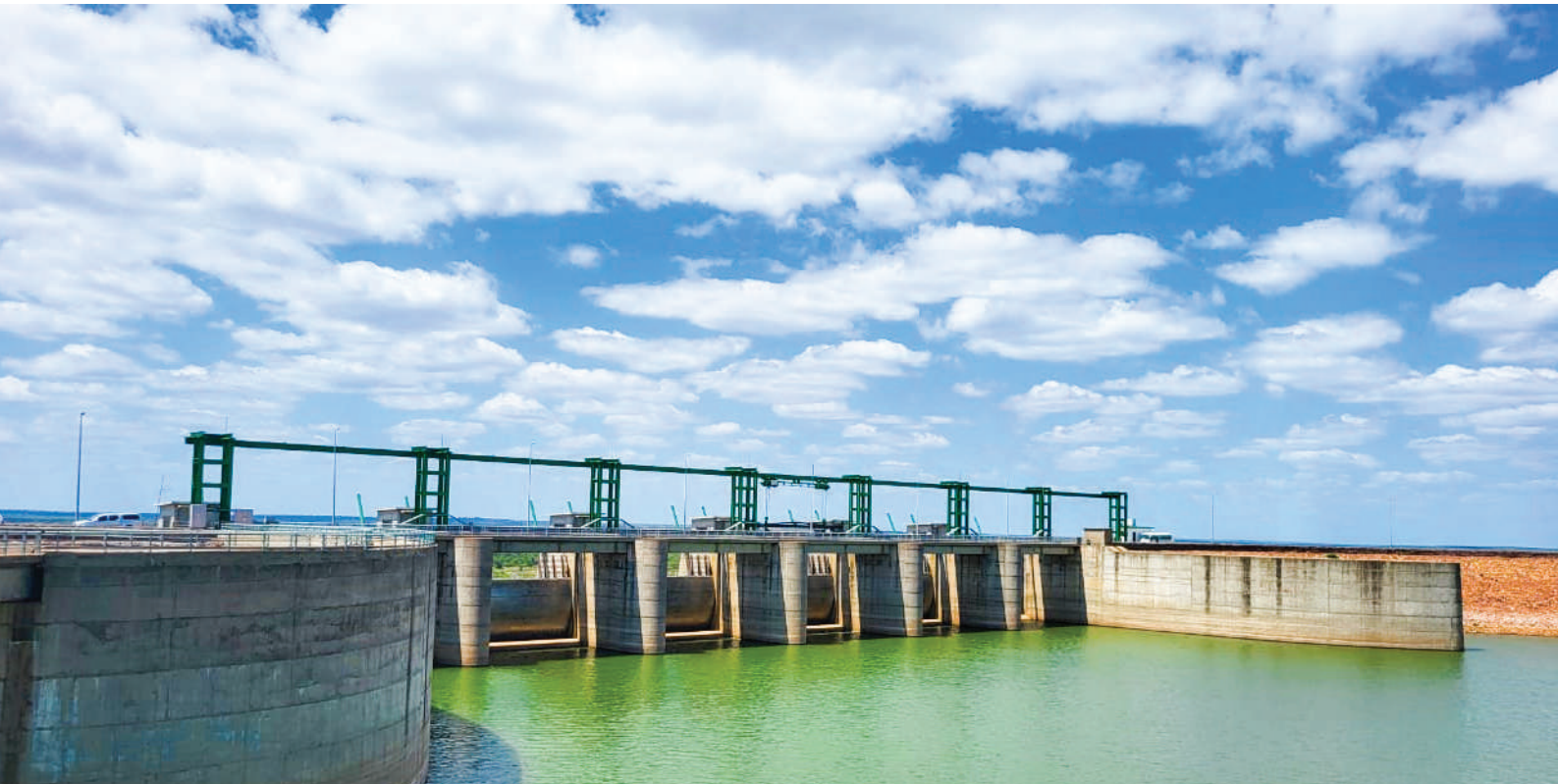
Dam Rehabilitation and Operational Recovery – Southern Mozambique
